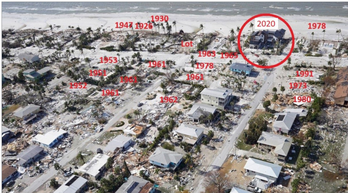
Image: Aerial photograph of Fort Myers Beach following hurricane Ian
